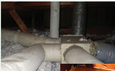
Top: Typical asbestos insulated ducting.
